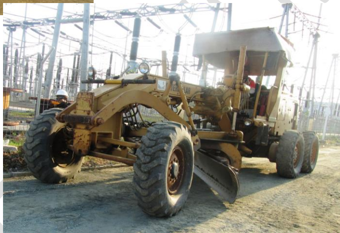
CATERPILLAR G140 in PLTU INDRAMAYU.
